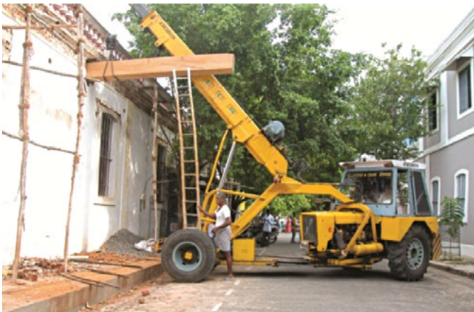
Expert assistance and techniques provided for restoration as part of the project
