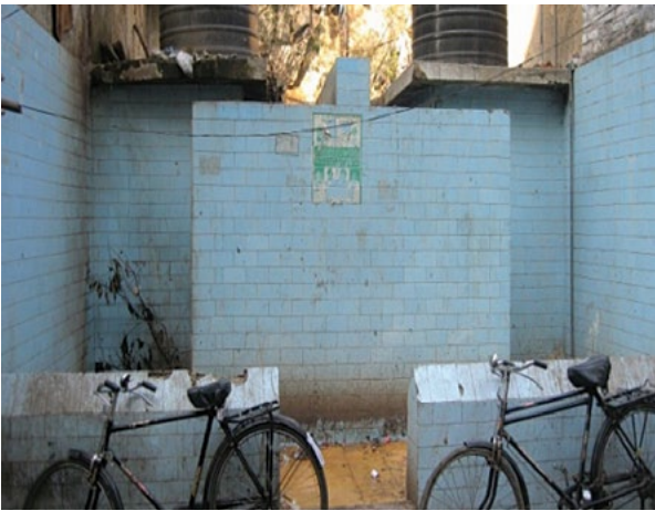
Upgradation of community toilet at Musafir Khana street
