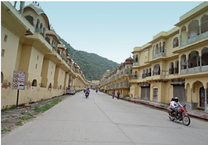
Ghat ki Guni: after restoration
